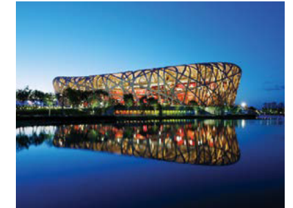
■ National Stadium (Bird's Nest)—Flame-resistance Cable
