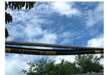
■ ICE-Figure-8 Self-supporting Cable
